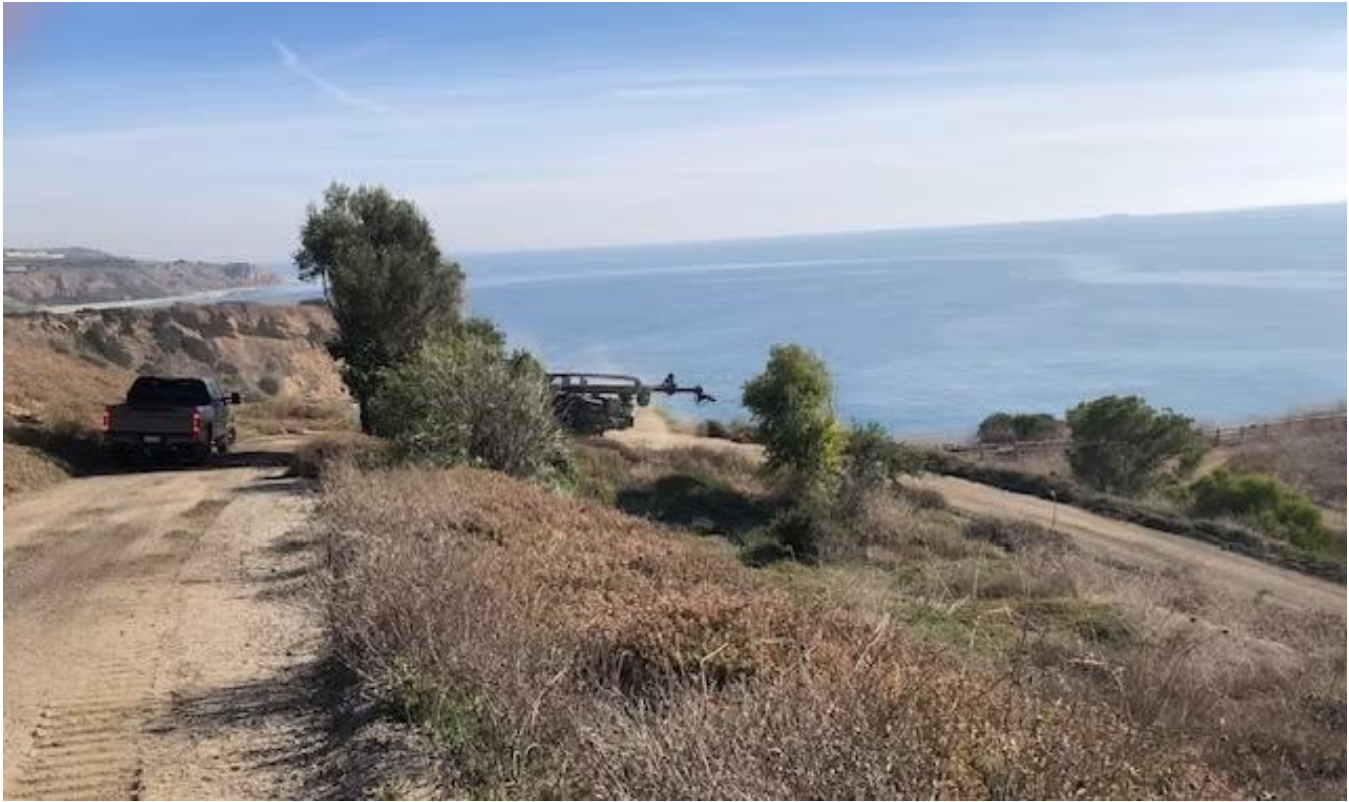
Figure 6-1 Abalone Cove Landslide Abatement District Drill Rig Arrival
